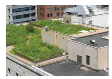
(Above Left and Right) The green roof on Chicago City Hall is over 70F cooler than nearby roofs on a summer day, as seen with a Forward Looking Infrared Radiometer. Source: U.S. EPA Reducing Urban Heat Islands: Compendium of Strategies<sup>#3</sup>
