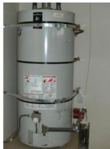
(Above) A hot water heater is strapped to the wall, securing its position in the event of an earthquake or major flood event. This increases the possibility that the appliance will not fall over and cause more damage or is damaged and needs to be replaced.
