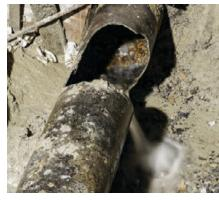
(Left) Old pipes corrode and break, causing system disruptions and local flooding.
