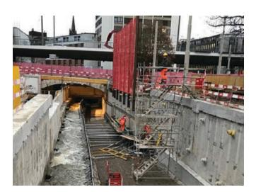
(Top Right) Retractable flood wall sectioning off a canal for repair work. Source: Aquafence
