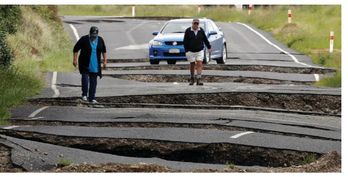
(Above) New Zealand residents approach an impassable roadway following a 7.5 magnitude earthquake in the region. This earthquake also caused landslides and soil liquefaction.
