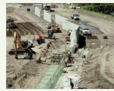
Installation of concrete form-work
