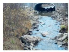
Rock Riffle Slows Water Flowing out of Culvert. Source: Frontier Environmental
