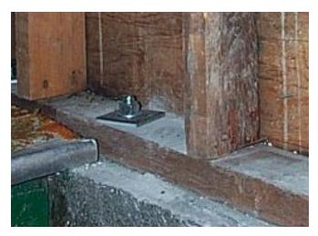
(Below) Foundation anchors help keep the building tethered to its foundation during a seismic event. Ideally they are coupled with a continuous perimeter foundation.
