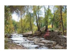
Rock Riffles Replace a Dam, Includes Stone Revetment. Source: City of Santa Fe
